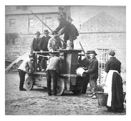
Manual fire pump dating from around 1720 in use. Note the large branch pipe on the top and the bucket chain water supply. It is thought this picture was taken whilst it was still in service in the 1880s!
