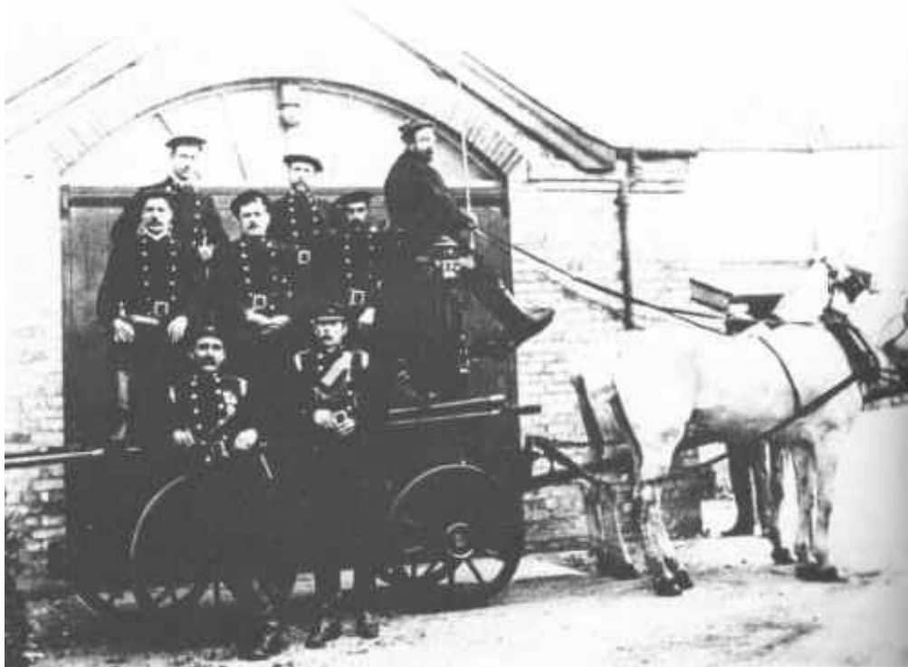
Captain Dix is shown standing in the front of this photograph (in the cap) of the Saffron Walden Fire Brigade outside their Depot at 3 Hill Street Saffron Walden
