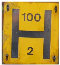
A modern standard hydrant plate, showing the diameter of the water main (in millimetres) in the top section and the distance the hydrant is from the plate (in metres) in the lower section.
